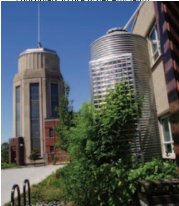
Water Tower and Rain Cistern, Chicago Center for Green Technology - Madison Environmental Group, Inc.
