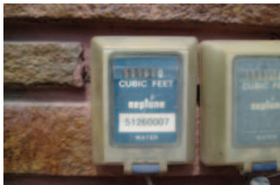
Water Meter - Madison Environmental Group, Inc.
