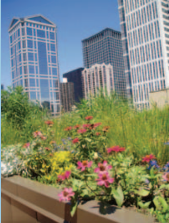
Chicago City Hall's Green Roof - Madison Environmental Group, Inc.
