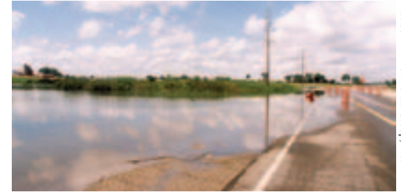
Flooded Highway, Central Wisconsin - Madison Environmental Group, Inc.
