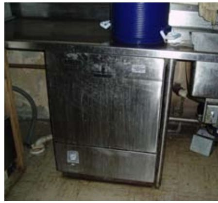
Hobart dishwasher with Hateo electric water booster
